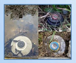
**Irrigation:** Sprinkler heads are not designed to be drip tight under backflow conditions.
