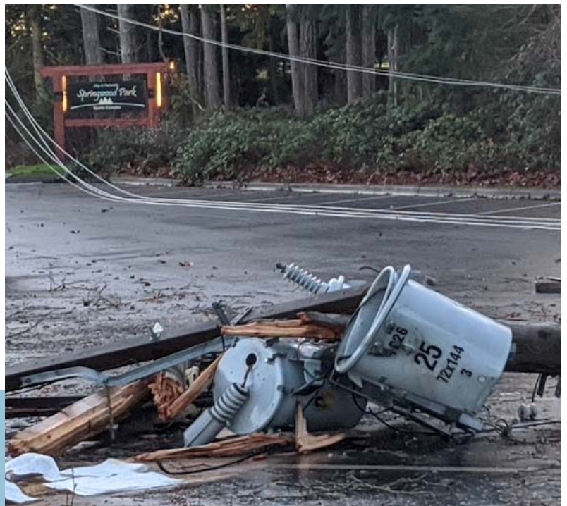
Power loss at Springwood Station due to a tree falling on power lines
