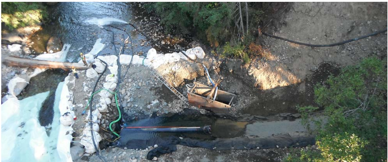
Water Treatment Plant Construction—River Crossing
