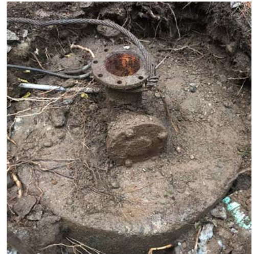
Abandonment of Springwood Well #4
