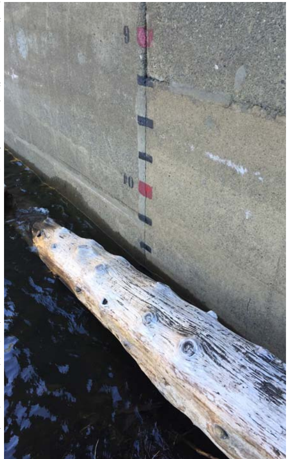
Arrowsmith Dam - two months of record breaking levels
