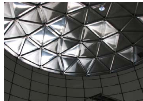
Inside of Reservoir #5
