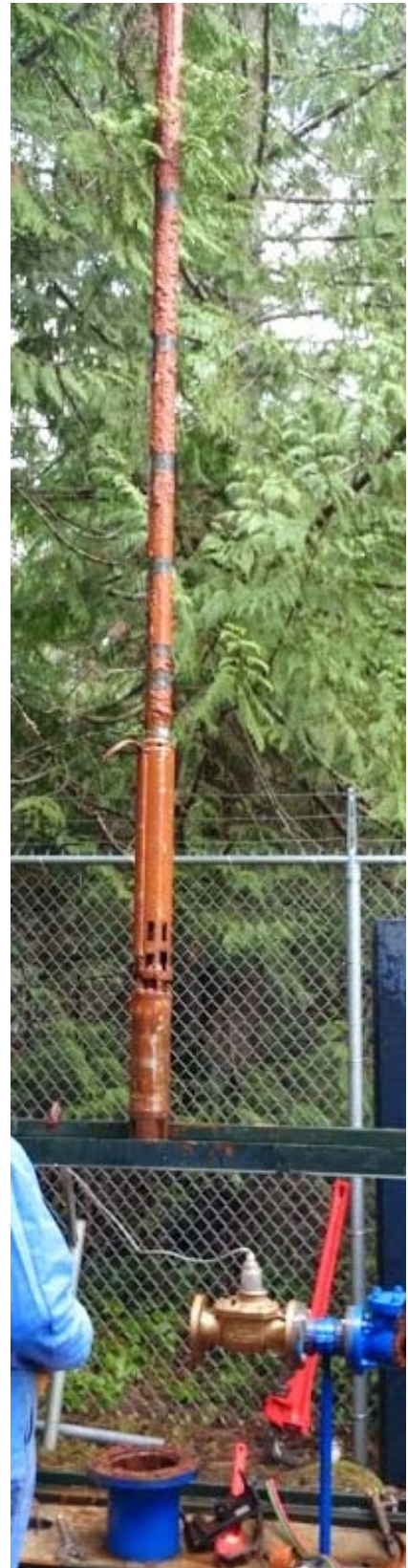
Railway Well being removed for repairs
