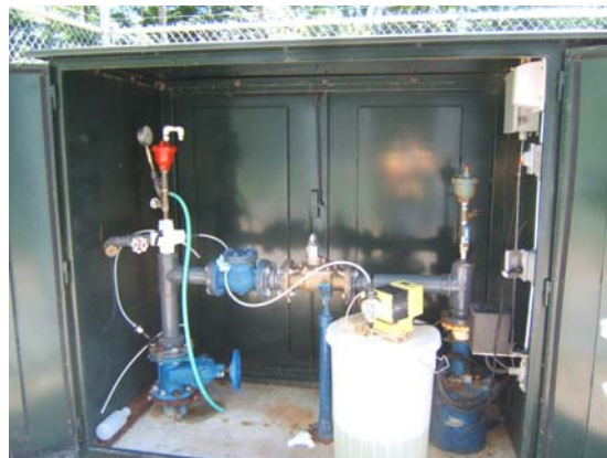
Railway Well Kiosk No. 5
